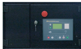
Deep Sea 7510 Loadshare Control Panel
